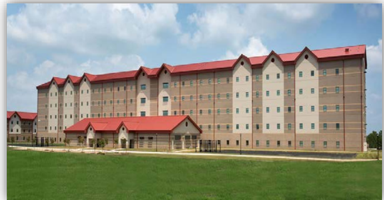
Advanced Individual Training Barracks Complex, Phase 2, Fort Gordon, GA
